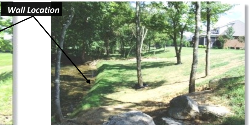
After the Flood
